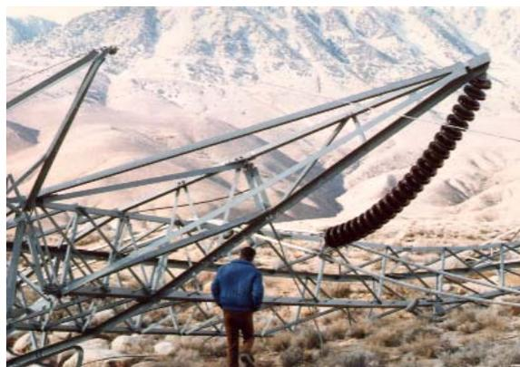
*Figure 1: One of 16 cascaded 500kV DC Towers collapsed at the Los Angeles Department of Water and Power (LADWP) in 1988 due to High Winds*
